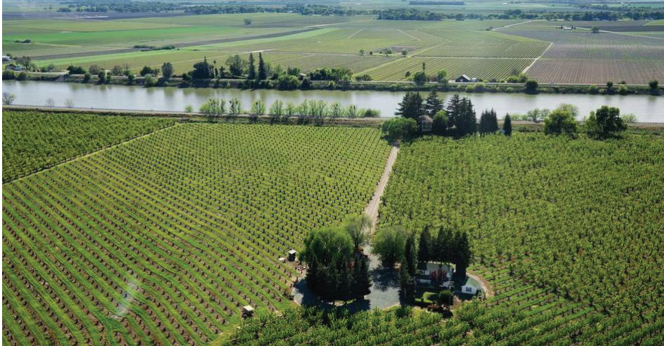
An aerial photo shows the region to be affected by the Delta water tunnels and intakes in the Courtland area. | Randall Benton rbenton@sacbee.comd
